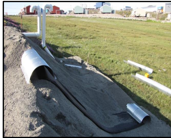
Heat drains structures at the Beaver Creek Test Site
