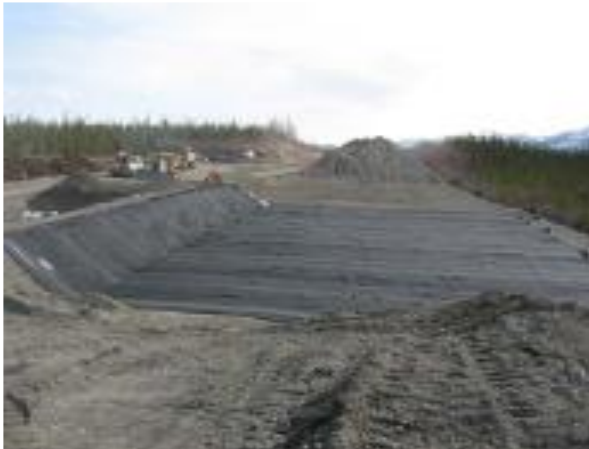
Heat drains structures at the Beaver Creek Test Site
