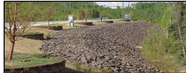
Air convection embankment uncovered, Beaver Creek experimental road site, Alaska Highway, Yukon (Guy Doré, 2010)
