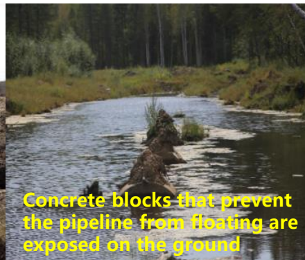
Pipeline submerged in water
