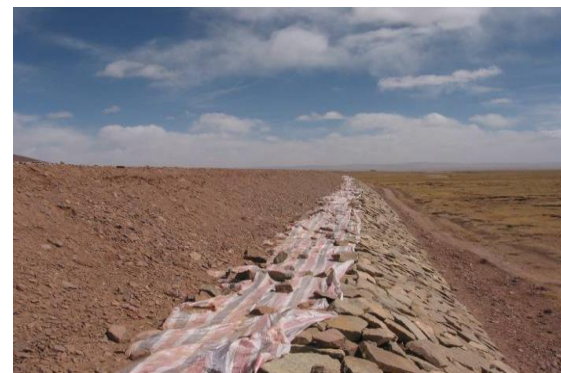
Air convection embankment uncovered, Beaver Creek experimental road site, Alaska Highway, Yukon (Guy Doré, 2010)
